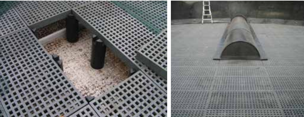
The assembled grating system installed in biofilter facilities
