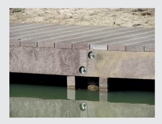
Substructures for boardwalks are made of either 8x23 cm or 8x16 cm profiles. Working with recycled plastic products is comparable to wood. The beams and piles are bolted together.
