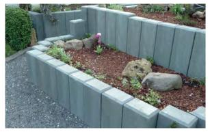
Round, rectangular or interlocking palisades offer diverse creative possibilities. They can be installed in straight lines or in curves. Graduations and height changes are possible without difficulty. With diameters of 6.0 to 20.0 cm, we have a suitable palisade for every application.
