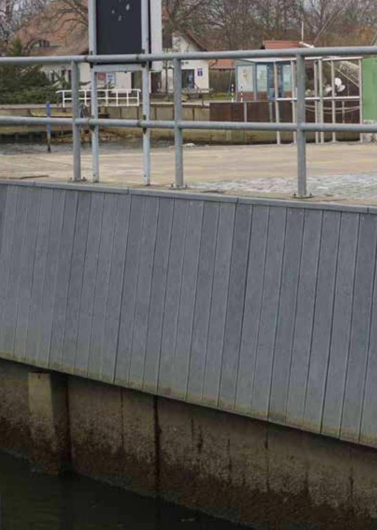
SHEET PILE WALL CLADDING WITH RUNNING BOARDS
